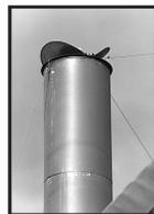
**Stack-in-a-Stack** - This design is based on the principle that rain falls at an angle. The inner stack is surrounded by an outer stack with space between the two. Rain runs down the inside wall of the outer stack, instead of down the inside wall of the inner stack and into the paint booth.
