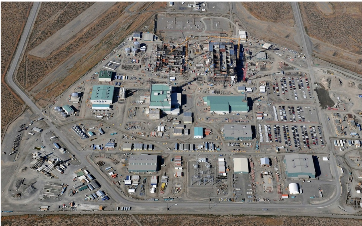
Aerial view of the WTP facility
