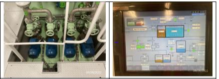
Photo #03 6/26/22 Image: IMG\_E1440 By: Dobrowski Description: Hamworthy Vacuum pumps Photo #04 6/26/22 Image: IMG\_E1445 By: Dobrowski Description: MSD Schematics Graywater, which includes accommodation and crew sink and shower water, galley water, laundry and possibly spa water is held treated using the 2<sup>nd</sup> Hamworthy bioreator and discharged outside of MOU related waters.
